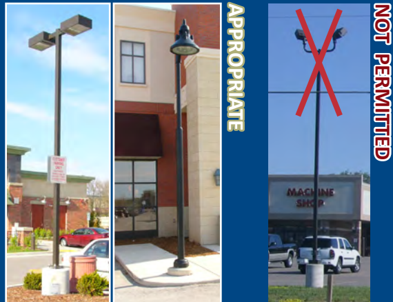
The two images on the left show good examples of low parking lot fixtures that project light only where it is needed, while the far right image shows an excessively tall light that is directed outward, creating glare and light trespass.
