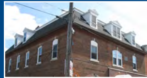
MANSARD ROOF (with dormers)
