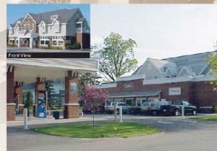
G Gas Station - 2nd Floor Office - Fuel Pumps in Back
